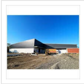
Warehousing Consultant Services
