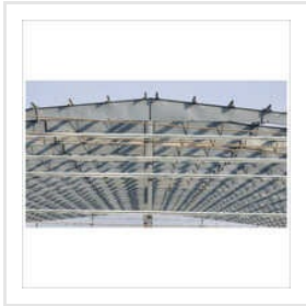
Warehouse Steel Structure
