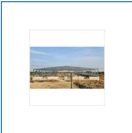
PEB STRUCTURAL SHED
