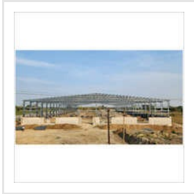
PEB Structural Shed
