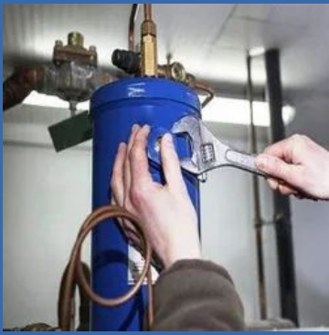
RO Plant Repairing Service
