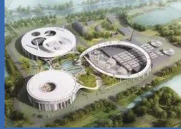
ETP Plant Services
