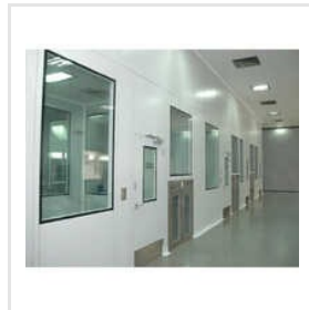
Modular Partition Clean Room
