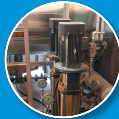
Closed Condensate System
