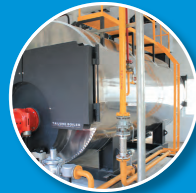
Constant Level Boiler Control
