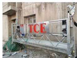
Rope Suspended Platform
