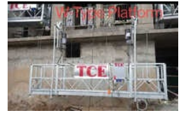
Temporary Suspending Scaffold
