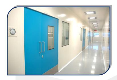
Intended to meets the particulars for Classes 100 to 100,000 (ISO 5 to ISO 8) condition. We are manufacturers, exporters and suppliers of clean room partitions with wall, puf panel and modular false ceiling in Ahmedabad India to worldwide with assured safety features. Clean Room puf Panels Consists of Following Sub Components: Clean Room Windows, Coving, Doors, 3D Corner Pieces, 2D Corner Pieces.
