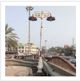
Street Lighting Pole
