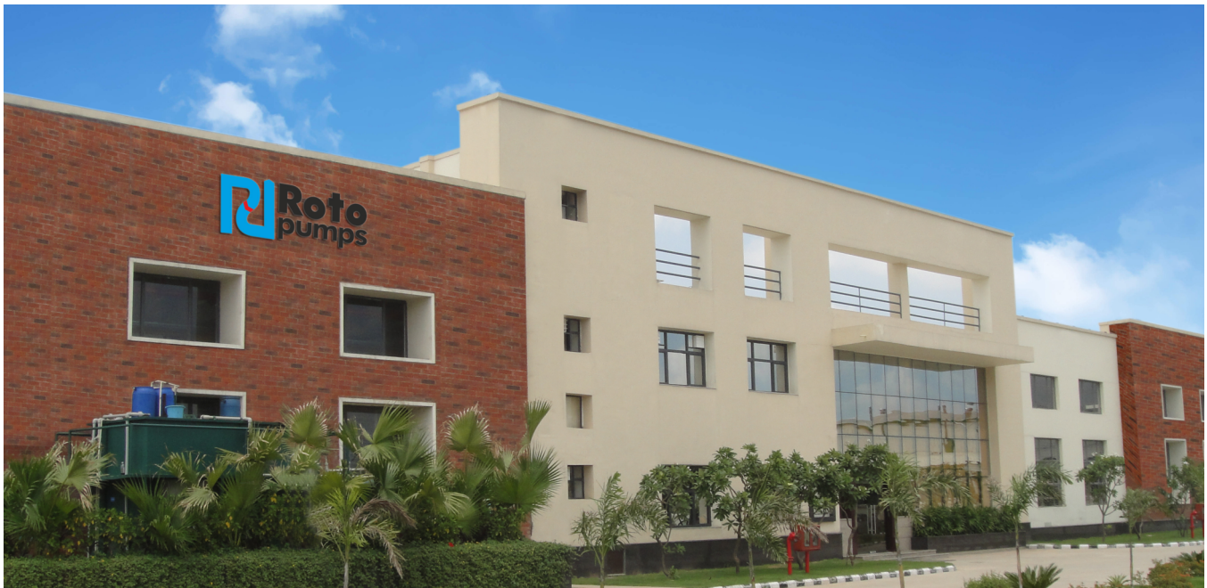
Roto Pumps Limited, Manufacturing Plant, India
