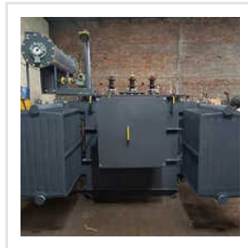
Three Phase Electrical Power Transformer
