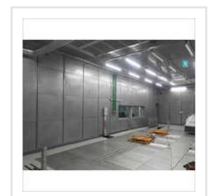
Acoustic Lining Walls
