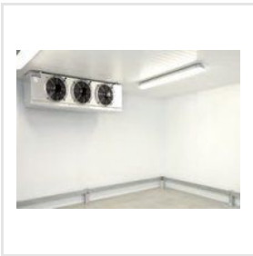
Walk In Chiller
