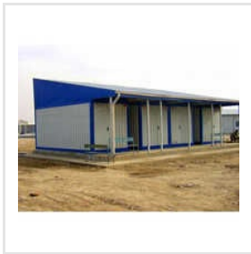
Pre Fabricated Room
