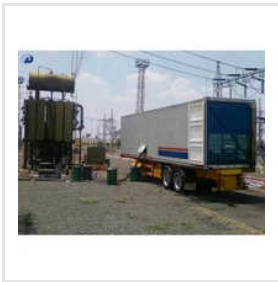
Automatic Oil Transformer
