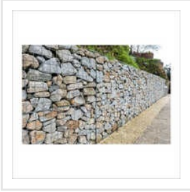
Stainless Steel Weldmesh Gabion Wall
