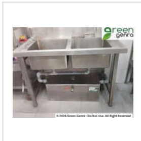
50 Ltr Kitchen Waste Water Grease Trap
