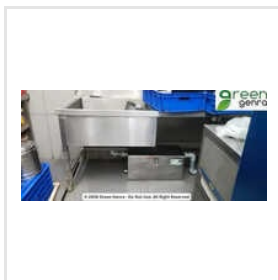
Stainless Steel Grease Trap
