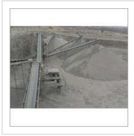
Sand Making Plant
