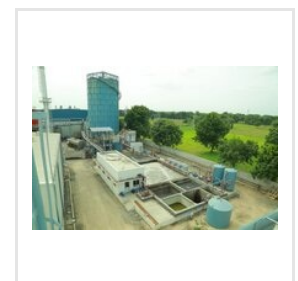
Effluent Treatment Plant
