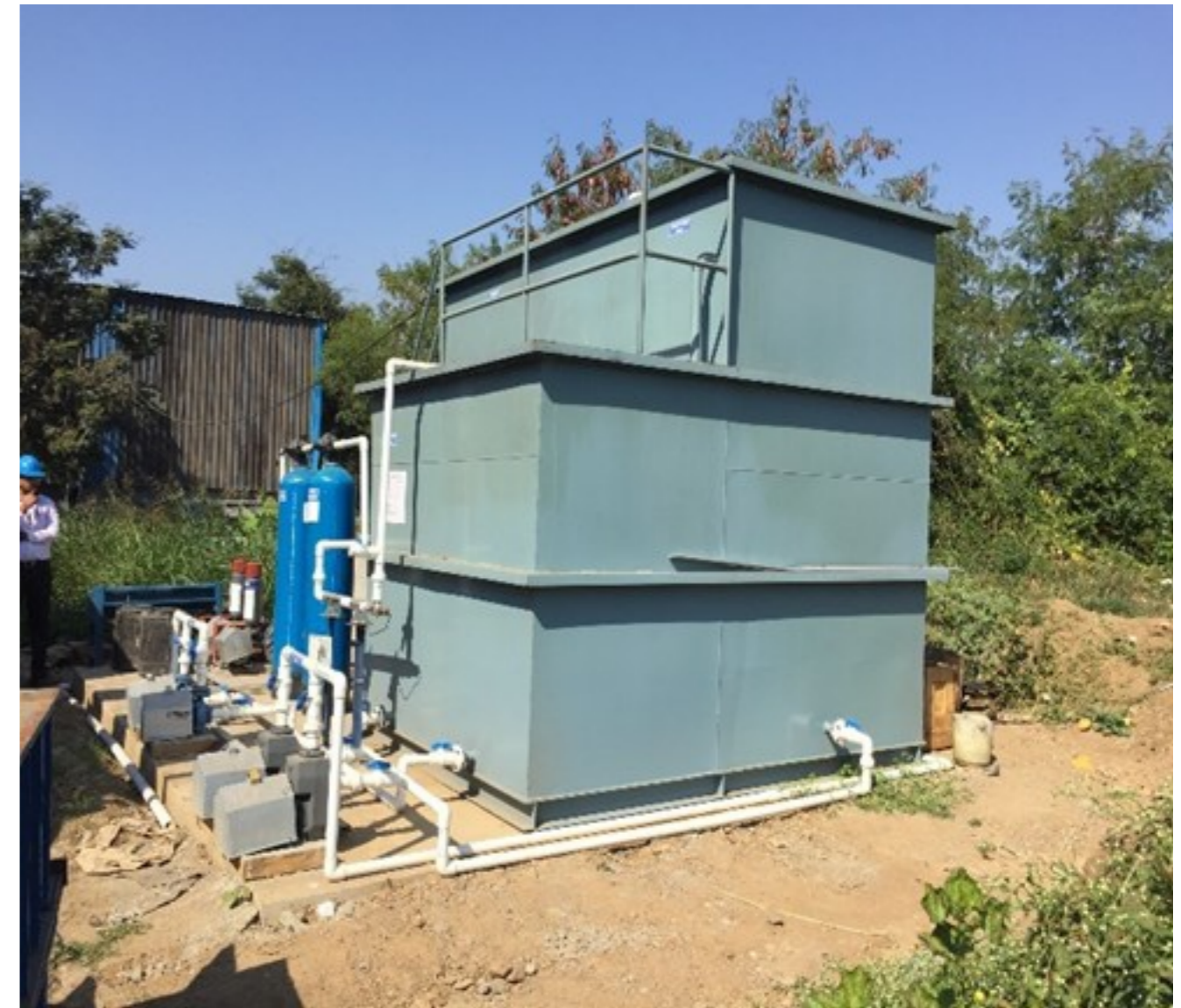
TYPICAL 40 KLD SEWAGE TREATMENT PLANT
