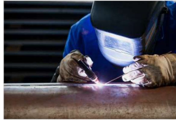
A man doing welding on stainless steel
