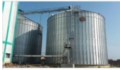
Grain Storage Silo
