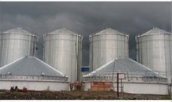
Industrial Storage Silo
