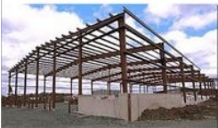
Pre Engineered Building Structure
