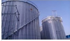
Paddy Storage Silo
