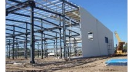
Prefab Steel Building Structure
