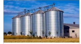
Rice Storage Silo
