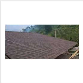
Sloped Roofing Shingles
