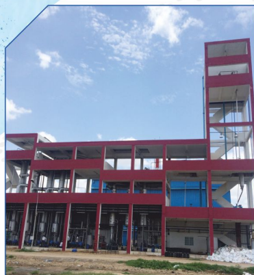
VANITEC CETP LTD 630 KLD
