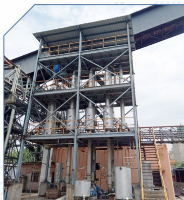
ACC CEMENT 60 KLD
