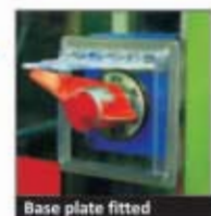
Base plate fitted
