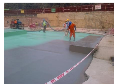
Fosroc Polyurea WPE application
