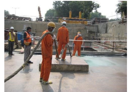
Spraying of first coat of Polyurea WPE
