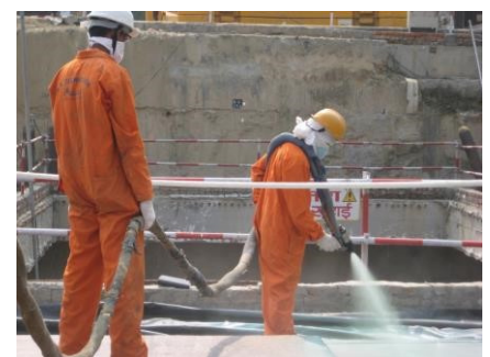
Spraying of Polyurea WPE on the station roof
