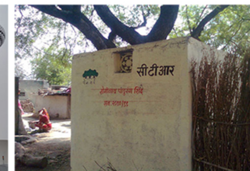
Construction of individual toilet
