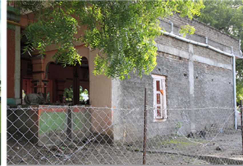
Roof top rainwater harvesting
