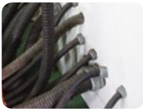
Outside the control panel
