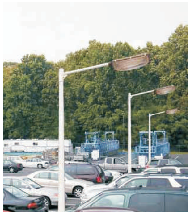
Parking Lighting Poles
