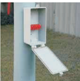
External Junction Box
