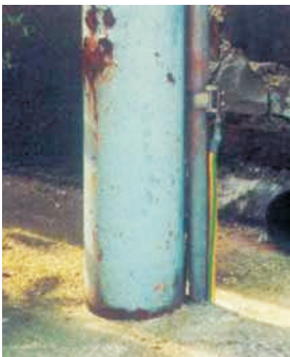
Rusted steel pole with required grounding
