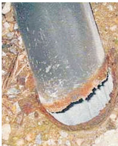
Weak Base of Steel Pole
