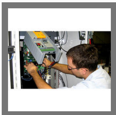
VFD Repair Services
